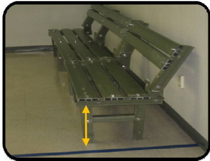
Fig. 7 – Optimal 18” Seat Height on the AOM EMTB
